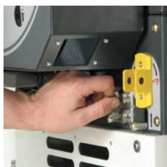
4- Lock the earthing switch by the key (if available)
