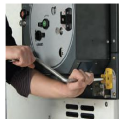
3- Open the earthing switch
