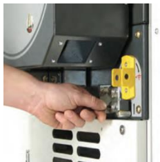
10- Lock the earthing switch by the key (if available)
