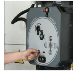
3- Unlock the air rotary isolator by the key (if available)
