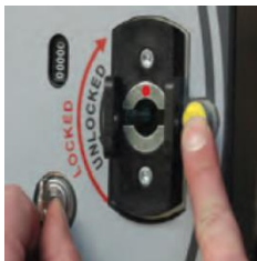
7A- Only in case of version equipped with key lock air isolator/earthing switch push the “yellow” button and free the key to fit into the earthing switch key lock
