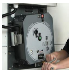
8- Lock the air rotary isolator in position “close”
