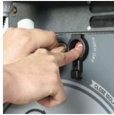
2- Lock the opening push button by the key (if available)
