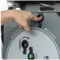
1- Open (OFF) the vacuum circuit-breaker
