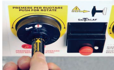
2.drawer in “disconnected” position
