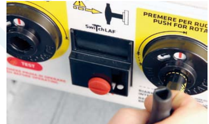
3.drawer in “connected” position
